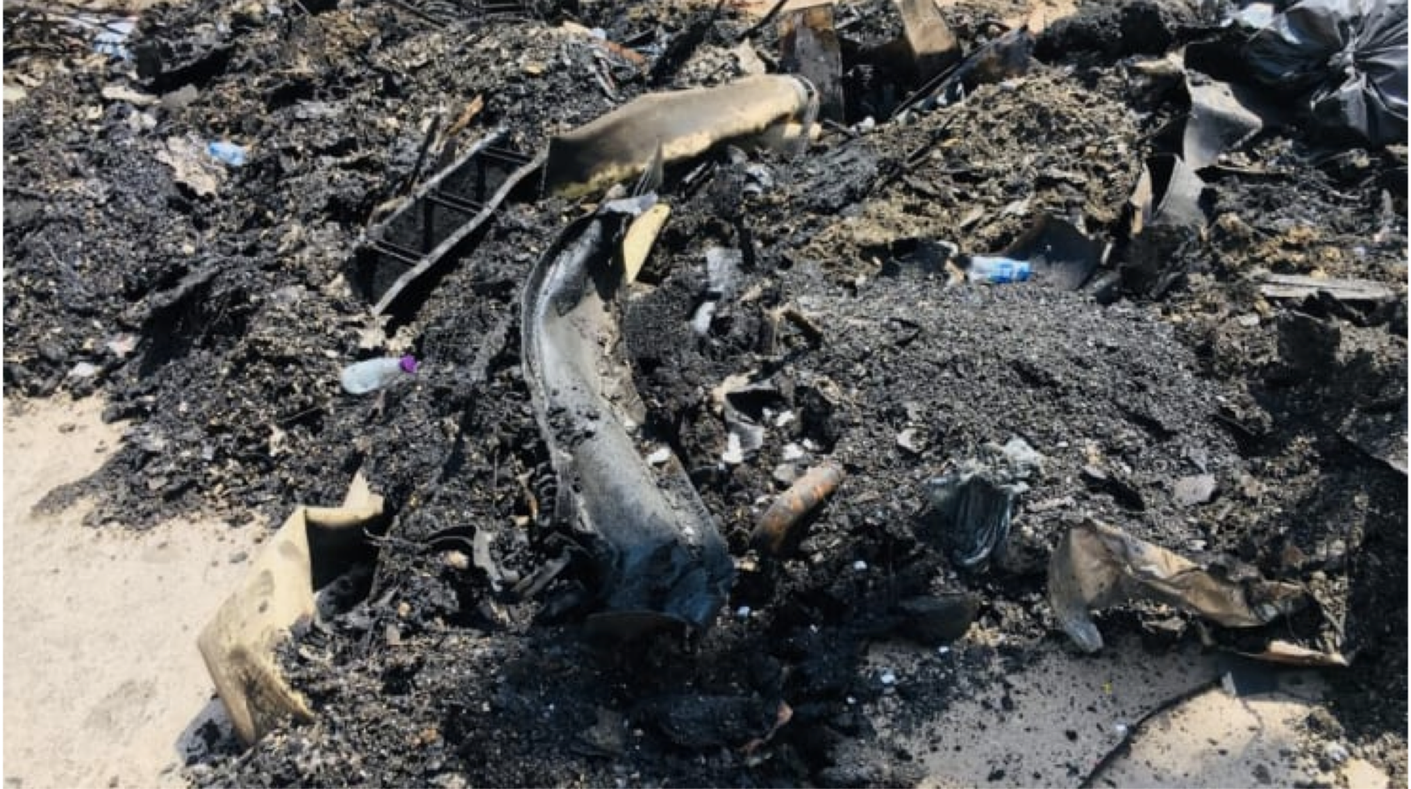
Debris at Saudi Arabia's Khurais oil processing plant following drone attacks, pictured on September 20, 2019.
