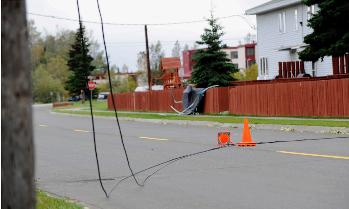
Figure 1. An example of a difficult pattern-recognition task for a computer: Downed power line. (Photo: U.S. Air Force/Tech. Sgt. Brian Ferguson.)
