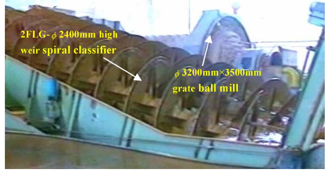
Fig. 9. Grinding units in the plant.
