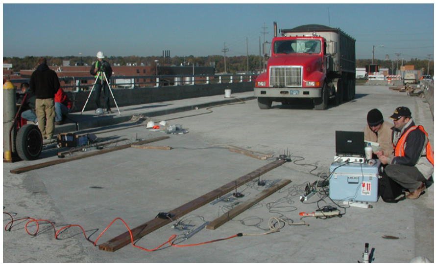
Michigan DOT field testing of engineered cementitious composite showed that the ECC link slab was even more resistant to deterioration than the concrete of the adjacent bridge decks while accommodating mechanical and environmental loads.
